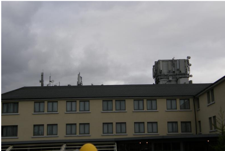
Transmitter Site Photo
